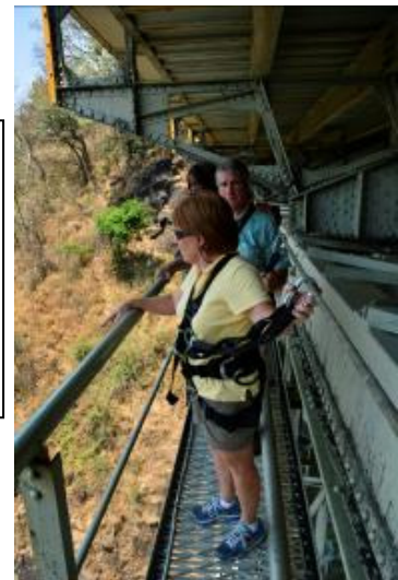
Chris and Gary shown hooked into harnesses on the catwalks that were used in the original construction of the bridge in 1904!
